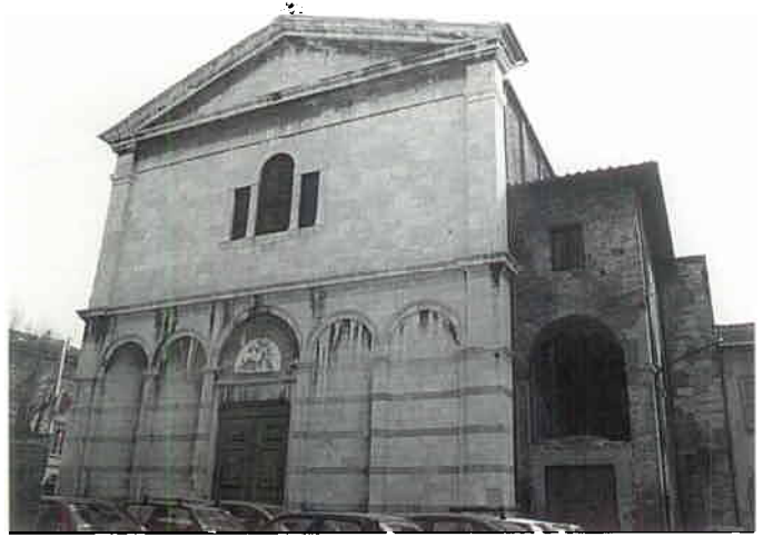
FIGURE 5. Facade of San Martino showing enclosed loggia and second-story room leading from choir to modern parish residence (photo, H. Flora).
